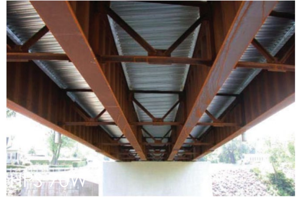
Girder bridge, Demonstration bridge in Bradford County, PA, USA
