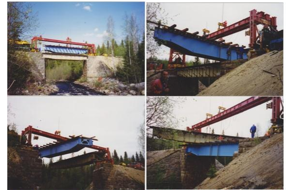
(i) new bridge transported to site, (ii) turning of bridge, (iii) switching of the bridges, (iv) new bridge in place and old bridge to be transported away.
